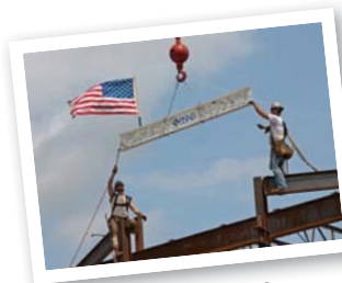
Construction on the Corporate Plaza began in 2010.
